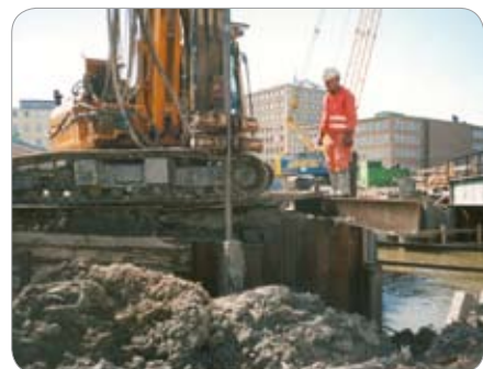
Göteborg – Sweden Foundations in water rich formation.
