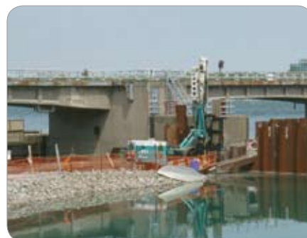
Niagara – Canada Construction of foundations for an 11 km long turbine tunnel.
