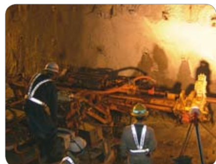
Chikushi tunnel – Japan Drilling of 200 m long horizontal survey holes.
